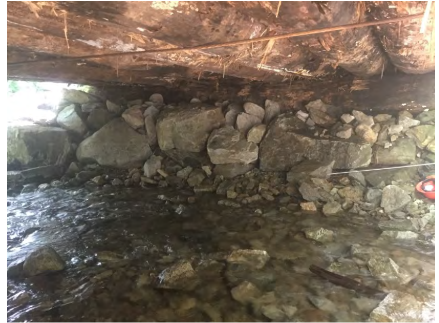
Right Bank Abutment when facing downstream
