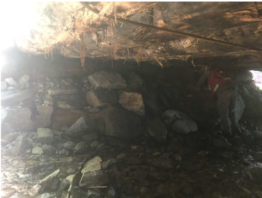
Left Bank Abutment when facing downstream
